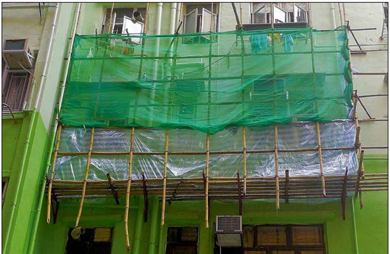
Truss-out bamboo scaffolding
