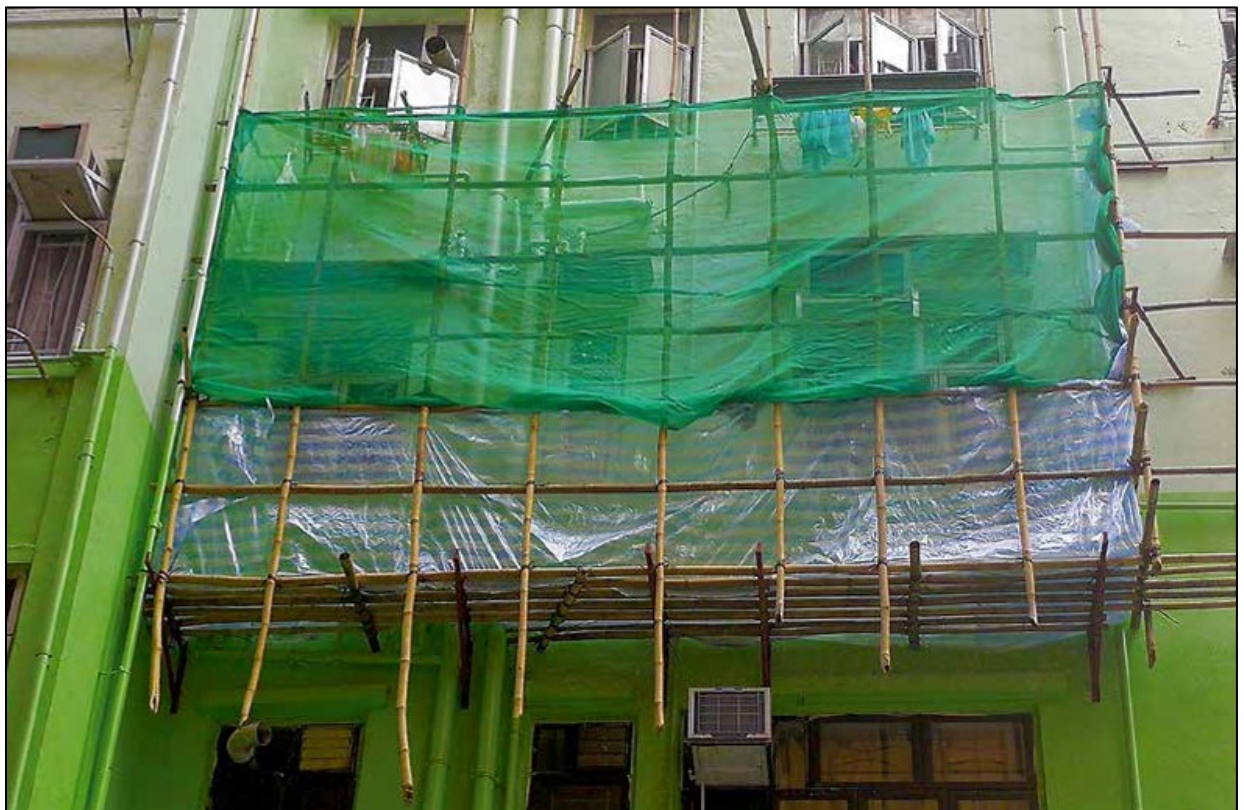
Truss-out bamboo scaffolding
